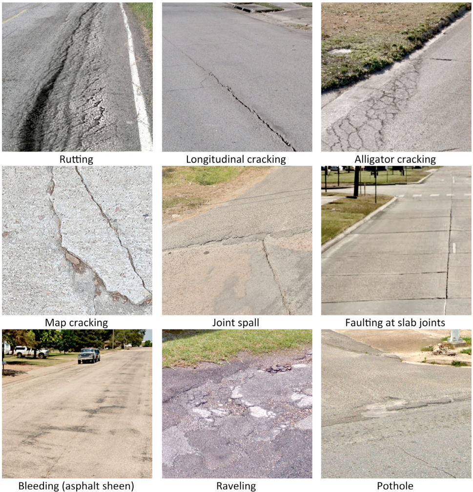
Fig. 4. Representative images of common pavement distresses observed in the dataset. Labels indicate the distress type. Photographs were captured by the research team during field surveys in Southeast Texas and illustrate typical manifestations of each distress type as classified in accordance with ASTM D6433 [1].
